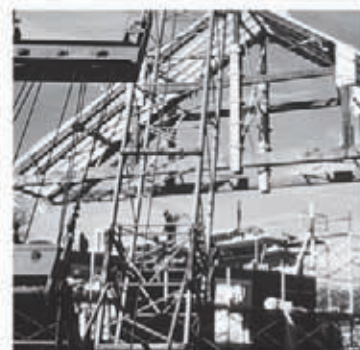
The 20x58 foot trusses from the 1812 Central Philadelphia Meetinghouse were moved to George School in 1973.
